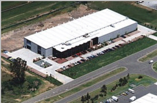
Above: Stage 1, Broens Industries 5800m 2 high-tech manufacturing facility at Williamson Road, Ingleburn
