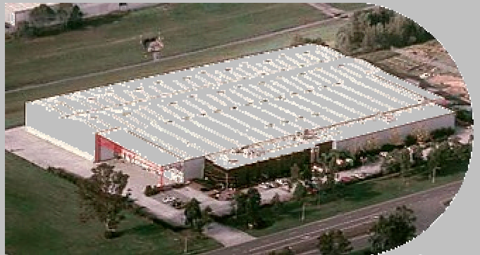
Above: Stage 2, Broens Industries 12,000m 2 manufacturing plant at Williamson Road, Ingleburn
